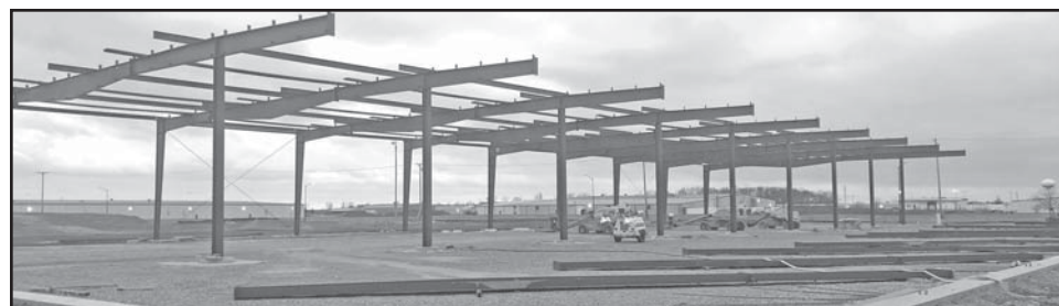
The initial steel erection for S&S Directional Boring's new facility
